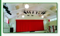
The hall suffered from sound reverberation and so we have had acoustic baffles installed to reduce the echo. All of the controls are accessible from the front of the stage so there is no necessity to take cables back to amplifiers or the projector. The new system with improved acoustics provides us with a near cinema-quality audiovisual system.
