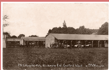
F.M.S Hospital Huts, Blackmore End
